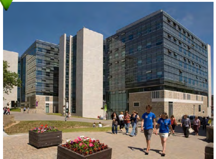
The Portland Square Building on the University of Plymouth campus, home of the new IODP 3 Science Office
